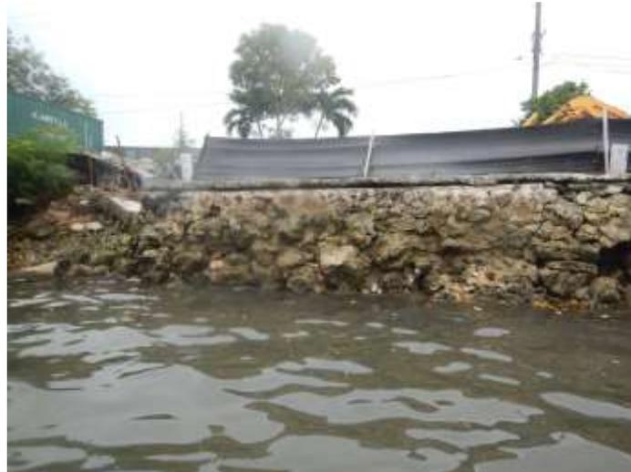
Figure 4. Ocean side of the Project site showing Silt Fence already installed, and a collapsed riprap wall.
